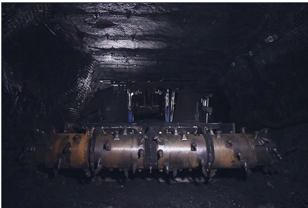
Fig. 14. Work site of bolter miner.
